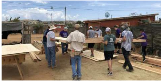
Building a home in Baja, Mexico - 2018
